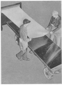
BLACK PAPER tape, available in widths up to 36 inches, protects smooth surfaces during outdoor storage up to six months in duration. The protective tape, shown in the photograph, is easily applied
