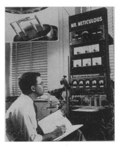
MAKES TRANSISTORS—"Mr. Meticulous," a robot device for assembling tiny experimental transistors, goes through its paces for Bell Telephone Laboratories' scientist R. P. Riesz. Inset shows a completed transistor compared with the edge of a dime. The wire shown is almost as thin as a human hair.
