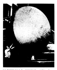
LIGHTNING SHIELD—This lensshaped steel tank, as part of one of the world's largest oil circuit breakers, will tame surges of electricity caused by lightning. Electric arcs during momentary interruption of flow of current are almost as hot as a nuclear explosion. The device is being manufactured in General Electric's High-Voltage Switchgear Department in Philadelphia.
