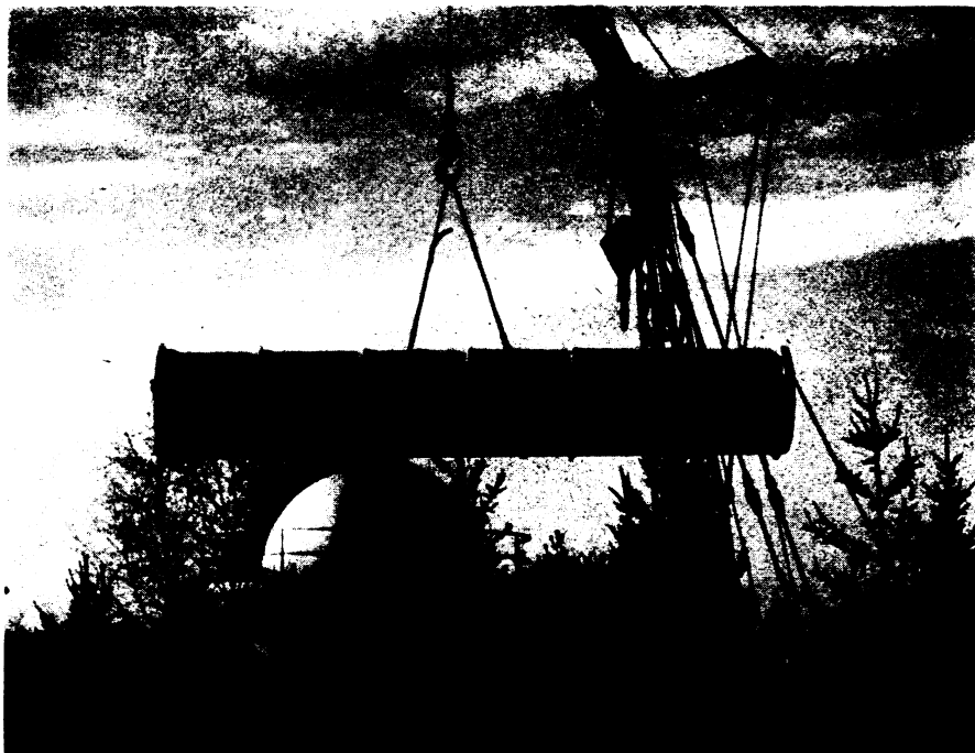
SPECTROGRAPH TUBE —Crane carries 52-foot-long cylinder for the giant spectrograph at the University of Michigan's McMath-Hulbert Observatory. The tube is four feet in diameter and will be a major part of the device to analyze the chemical composition of the sun.
