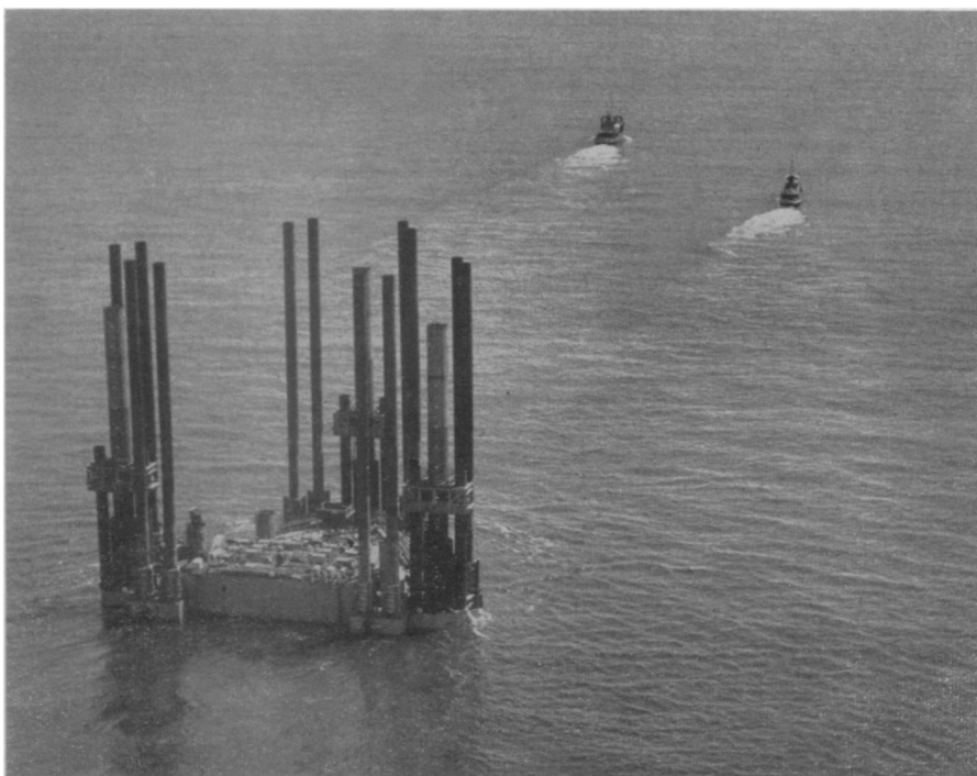
ATLANTIC RADAR WARNING —Two ocean tugs tow the 6,000-ton "Texas towers" that will become the first of a series of offshore radar stations in the United States continental defense system. Tugs of Moran Towing & Transportation Co., Inc. are shown moving the structure out of Boston harbor on its way to permanent location at George's Bank, 100-odd miles off the New England coast.
