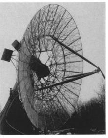
BIG "DISH"—The 60-foot radio telescope at Harvard College Observatory, recently dedicated, can rotate to focus on any part of sky and can tilt at the same time. Built to collect radio waves from space, the saucer-shaped receiver is largest of its kind in the country.
