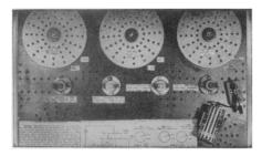
This is the control panel of GENIAC set up to solve a problem in symbolic logic analysis.
