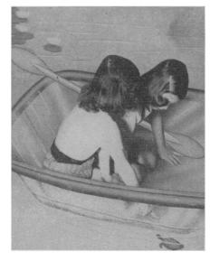
48 inches long, 10 inches deep and 32 inches wide. Molded in one piece, the leakproof boat is built to stay afloat even when full of water. It can carry 250 pounds.
