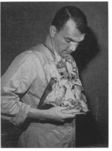
AUTOMATIC INFLATOR — Expected to become a standard safety feature for life jackets is this device that automatically inflates a pilot's "Mae West" within 15 seconds after immersion in water. George Smith, test pilot at North American Aviation, Inc., demonstrates position of the lifesaving device.
