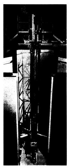
TALL TOWER—The core of the reactor Battelle Memorial Institute now operates is located at the bottom of this suspension tower. When sufficient fuel elements are in their proper positions, fission produces gamma rays and neutrons for use in research. Tubes entering from the sides of the pool have samples for irradiation inside them when the reactor is operating.
