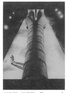
SILENT NIGHT—To meet the around-the-clock problem of testing tomorrow's powerful jet engines without disturbing nearby residents, the British firm of de Havilland has designed at Hatfield, Hertfordshire, England, a testbed fitted with a silencer that can handle engines of more than 30,000-pound thrust. A low-pitched rumble and the shimmering of exhaust gas are the only signs of the tests.
