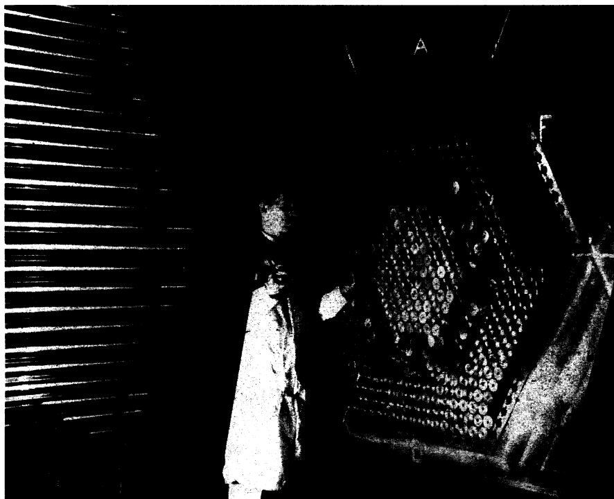
ATOMIC HONEYCOMB —A technician inserts a fuel rod into the preliminary pile assembly at the Knolls Atomic Power Laboratory. The reactor, first to be operated in the northeastern United States, is believed to have set a record in that it has been started up more than 10,000 times in experiments carried out on reactor designs.
