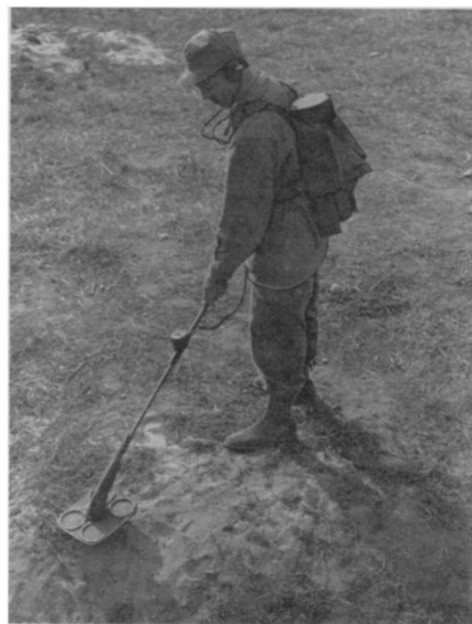
MINE DETECTOR —This is "Polly Smith," a metallic mine detector used in Korea. Its grandfather, and the first of all mine detectors, was invented by an amateur. Now the Government needs a mine detector that can locate non-metallic mines.
