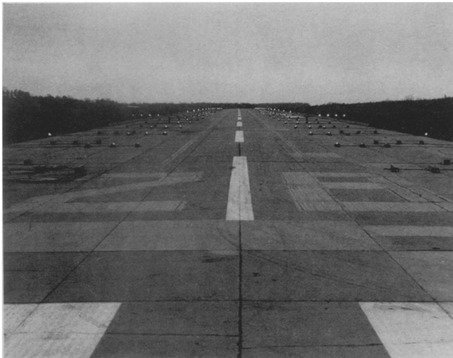
ELIMINATING "BLACK PIT" —Special boxes which contain experimental lighting elements are shown in this daylight photograph at Andrews Air Force Base. The lights are being tested in a program to provide for safe night landings.
