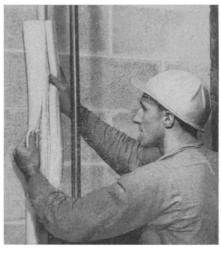
has a service range of from minus 200 to 250 degrees Fahrenheit. The snap-on material, shown in the photograph, available in almost any size, shape and thickness, can be stretched to nearly twice its original size, and will not support combustion.
