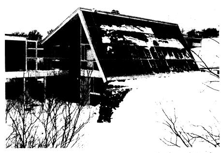
SOLAR HOUSE—A snow-swept view of the first solar house designed to meet modern living requirements in a northern climate shows part of the mechanism for "catching" the sun's heat. At the right is the glass-faced solar collector that forms all the visible south side of the house. At the extreme left is part of the screened porch that provides outdoor living space for the second-story living room. The house is seen from the southwest.
