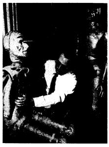
ANTHROPOMORPHS — Rubber skinned dummies that conform to the shape, size and weight of human pilots are used by North American Aviation engineers in perfecting systems for saving pilots' lives. Electronic equipment in chest and stomach cavities records important information.
