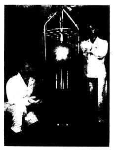
ITALIAN REACTOR—Technicians of Atomics International, North American Aviation, Inc., fit precision milled graphite reflector blocks around the "core" of the 50-kilowatt nuclear research reactor being built for the Enrico Fermi Nuclear Study Center in Milan, Italy. The core, which will contain uranium in a water solution as fuel, is upside down for easier assembly. The reactor will be used for research and training in nuclear and associated fields.
