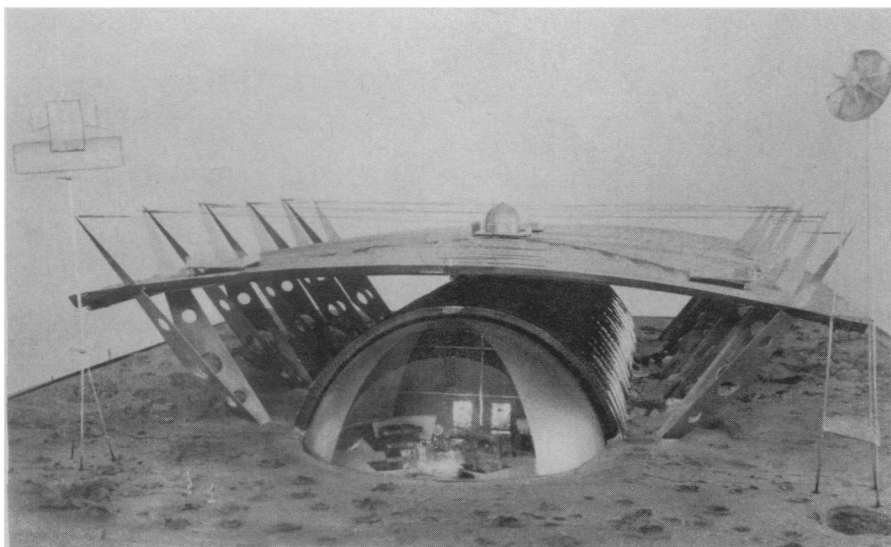
MOON HOUSE —A detailed five-by-six-foot scale model of the moon building designed and engineered under the direction of Dr. John S. Rinehart shows the plastic observation bubble and the slightly curved meteorite shield above the roof. It would be constructed of aluminum alloys.
