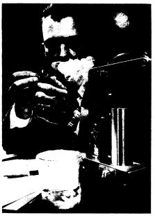
WARNING TUBE—An ultravioletsensitive tube that responds to flame, smoke and combustible vapors simultaneously indicates the presence of any of the three. Mathias J. Grundtner, a research scientist with the Minneapolis-Honeywell Regulator Company, demonstrates how the tube works when both fire, smoke and combustible gases (in the beaker) are present. The four-inch tube "sees" invisible ultraviolet light.
