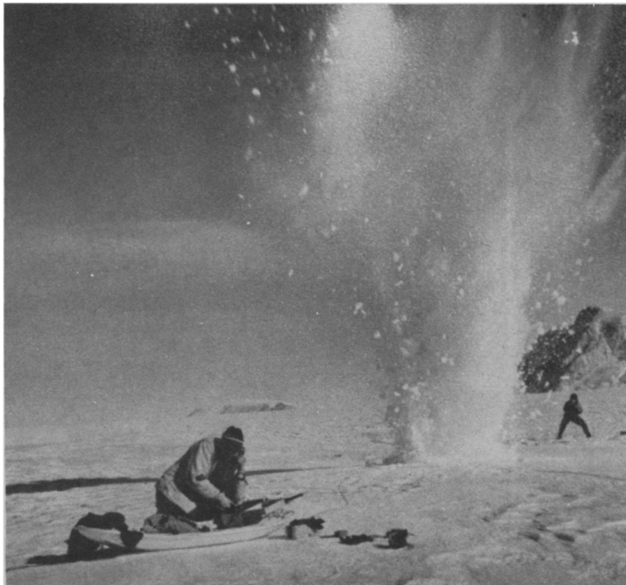
SEISMIC EXPLOSION —Ice thickness is measured along an antarctic traverse by using an explosion.
