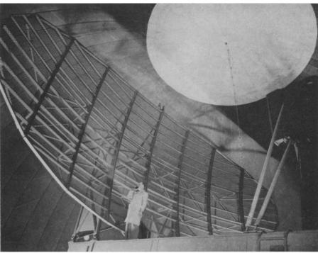
HIGH POWER RADAR—A "super power" radar that detects air target at far greater ranges and at higher altitudes than present-day air defense radars has been developed by the General Electric Company jointly with the Air Research and Development Command. The upper photograph shows technicians installing a multi-million watt Klystron tube that permits generation of extremely high powers in the microwave region. The feed born, antenna and 50-foot rubberized radome are shown below.
