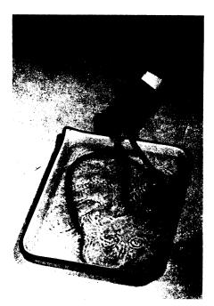
ELECTRIC "EEL"—A snake-like assembly of tiny battery cells that can be wound on a drum along with the cable, is activated when unreeled into water. Rubber rings separate silver chloride links from zinc segments. Developed for the U.S. Army Signal Corps by Aerojet-General Corporation, Azusa, Calif., the snake batteries are spliced into cable every mile to boost voice or teletypewriter signals.
