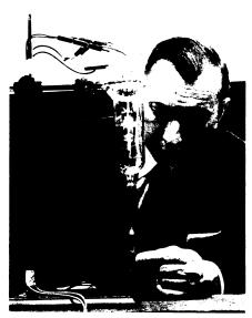
POTENTIAL POWER—This experimental thermionic tube has a glowing wire that emits electrons, making a current flow in ionized cesium gas. The cesium capsule at the bottom of the tube is pointed out by Dr. J. W. Coltman of Westinghouse Electric Corporation, where therminic power generation is under development. Thermionic devices may be used for space power or to add extra power to nuclear generating stations.
