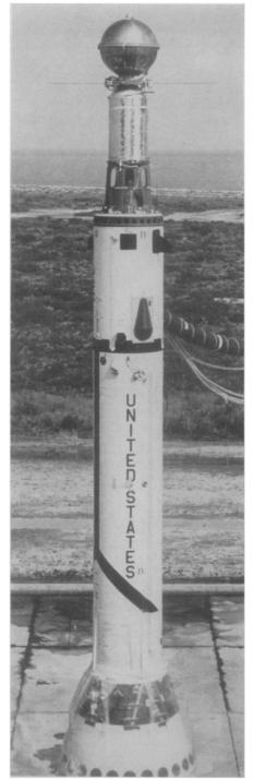
ROCKET WITH ECHO—The 28inch canister on top of the Delta
