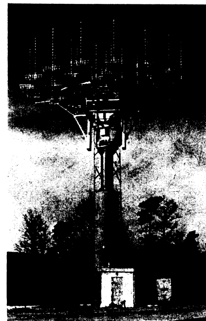
END-FIRE ANTENNA —will record telemetry from rockets tested at NASA's space flight station, Wallops Island, Va. It was built by General Bronze Corp., Garden City, N. Y.
