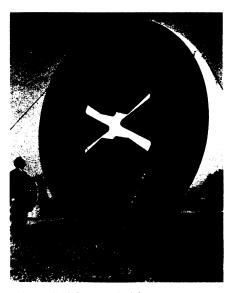
FOR SPACE BOOST—A cross section of a 14-foot diameter rocket motor that would total 63 feet in length. The solid propellant motor is under study for the National Aeronautics and Space Administration at the Thiokol Chemical Corporation, Trenton, N. J. Seven full size motors could power the first stage of space vehicles.
