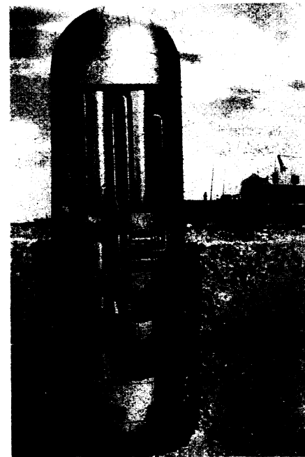
GERMAN ATOM PLANT —The first German atom power plant has been opened near Frankfurt on the Main. The reactor as well as the action primary circuit is built into the cylinder.
