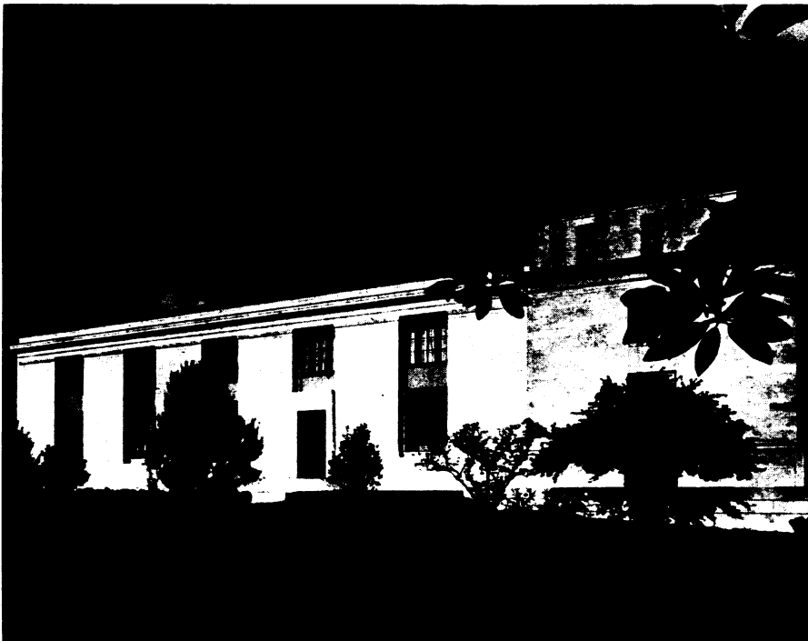
HALL OF LIFE SCIENCES —The new west wing to the National Academy of Sciences, just completed, stands sedately in beautiful surroundings.
