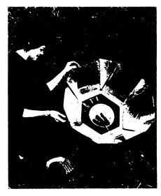
SOLAR STOVE, shown in the photograph, requiring no fuel but the sun will be ideal for picnicking and for persons in developing countries when put on the market. Made of a hexagonal cardboard box with aluminum foil reflectors, the stove is capable of heating a quart of soup to 175 degrees Fahrenheit in less than 35 minutes on a sunny day. The interior of the box, insulated and lined with black foil, forms the oven.
