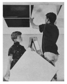
installation in the home is suitable for lowering ceilings, for hiding bad plaster, wiring, pipes and ducts, or for adding fresh beauty to the home. No special skills or tools are required to assemble the system. Its lay-in ceiling panels, cut in convenient 2x2-feet and 2x4-feet sizes, come in acoustical, decorative and translucent styles. Moulding, cross trees, hanger wires and other components are available along with the panels.
