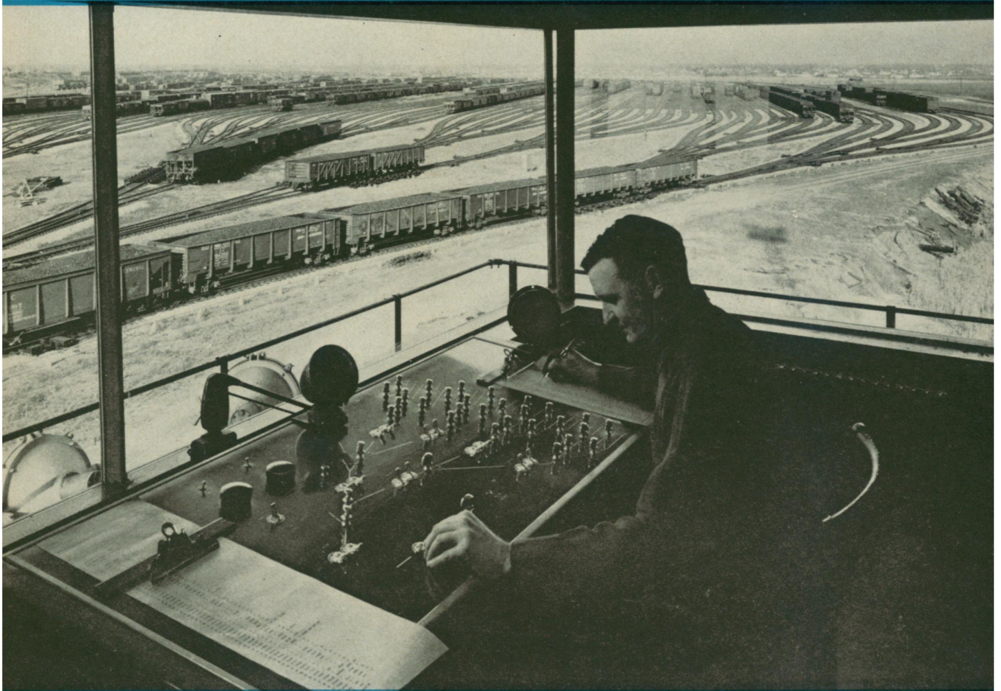
Illinois Central Railroad
