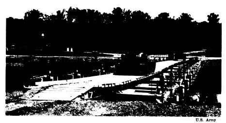
MOBILE FLOATING ASSAULT BRIDGE—A 334-foot span consisting of ten interior and two ramp bays of the mobile floating assault bridge supports a 47-ton tank and a 19-ton armored personnel carrier in tests at Fort Belvoir, Va. The bridge was erected in about 25 minutes by 36 men.
