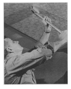
ceiling like wallpaper for installation. The heating element consists of panels of a flexible "sandwich" of two outer layers of thin vinyl and thread-thin resistance wiring interwoven with nylon net. Plugged into regular household electrical outlet, the system emits waves of radiant energy distributing heat evenly throughout the room. Each has its own thermostatic control.
