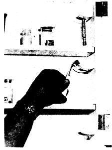
SAFETY RAZOR HOLDER, shown in photograph, will keep a safety razor safely out of the way, yet readily available. The holder made of plastic can be mounted permanently on any surface, inside the medicine cabinet or on the wall. The holder is scoop-shaped with a slot for the arm of the razor. An extra holder could serve as a convenient storage place for blades.
