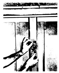
ALUMINUM FOIL TAPE, shown in photograph, comes in rolls and is useful for patching leaky downspouts, gutters, garbage pails, drainboards or air conditioning metalwork. The pressure-sensitive tape is applied after the area around the hole is cleaned with fine steel wool. The amount of tape necessary is cut off, firmly pressed down with a blunt tool over the area to be patched and then smoothed out to produce a weather-proof and long-lasting repair.
