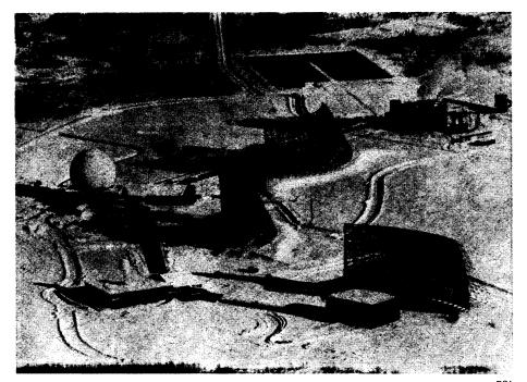
ELECTRONIC EYES-A giant tracking radar designed and built by Radio Corporation of America has been placed into operation at the Ballistic Missile Early Warning System site at Clear, Alaska, by the U.S. Air Force. The tracking radar, housed in a radome made of paper, fiberglass and plastic, will provide long-range, ultra-high-speed warning in event of a ballistic missile attack over the top of the world.
