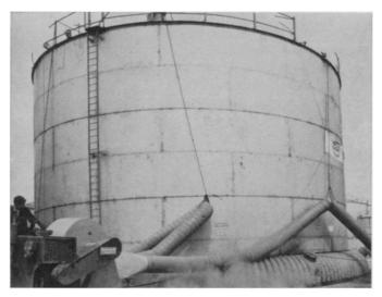
The use of air cushion avoids the need for careful preparation required for conventional methods where the tank is moved on rollers or bogies.
