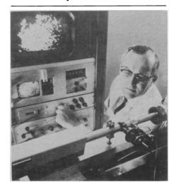
Flexibility is the word to describe a metallurgical research tool that can also be used for such diverse functions as counting cancer cells, bacteria, mineral and powder grains, air pollutants, and determining the sizes and shapes of pigments and particles that make up plastic and paint.
