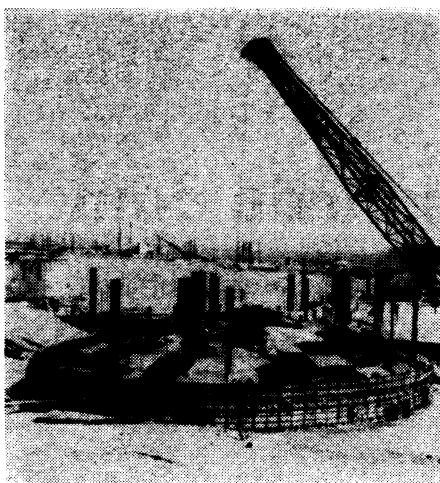
AEC Waste tank: Storage, not disposal.
