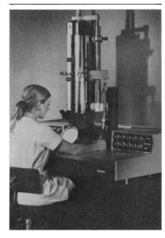
the inexperienced operator, Philips Electronic Instruments has developed an electron microscope that will produce images with a guaranteed resolution of 9 angstroms, simply and rapidly. The Model EM 201 gives the operator an unobstructed view of the main 4.7-inch diameter fluorescent screen through a 5.5-inch diameter window.
