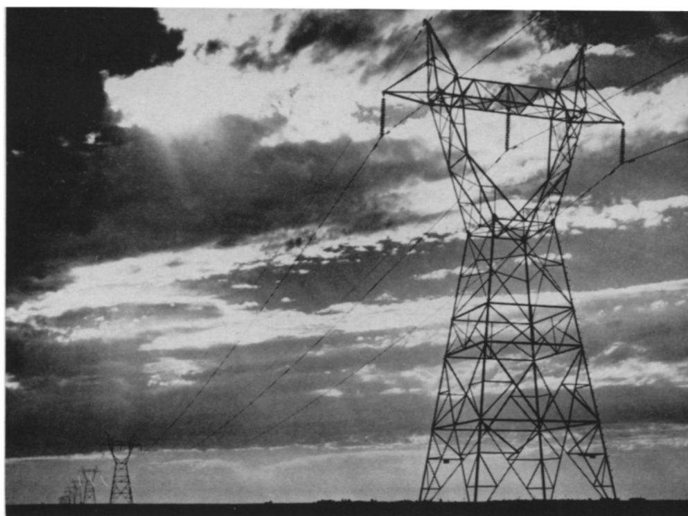
Bureau of Reclamation
