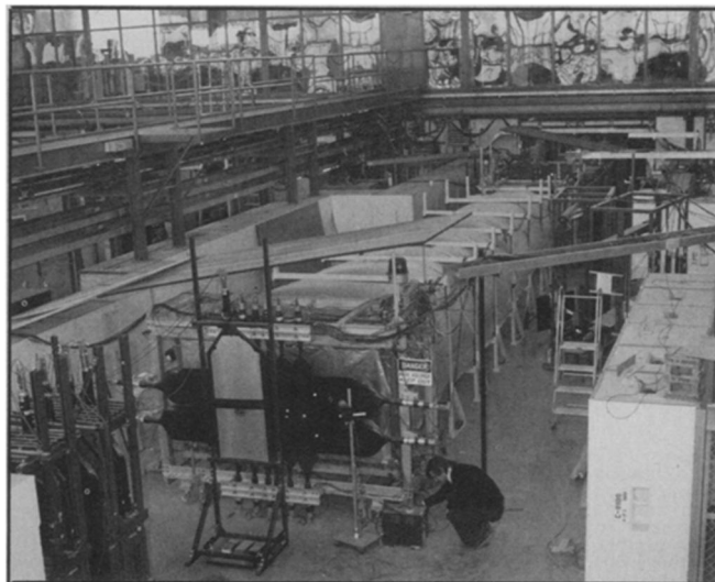
Crossed arrays of hodoscopes are the most conspicuous elements in this experimental setup on the floor of FermiLab's meson building.
