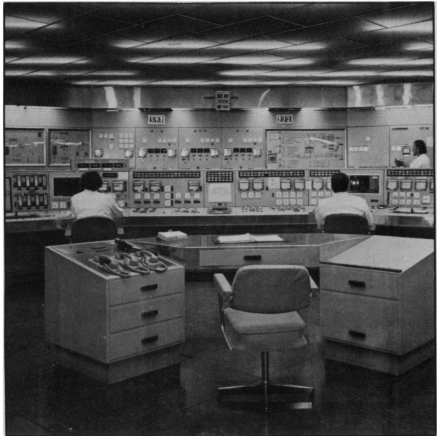
Operators sit at computerized control panel of the French Phénix breeder reactor.
