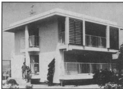
Collectors on terrace of solar house.
