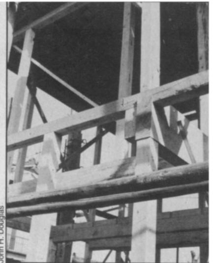
Intricately carved beam ends are still used in typical Japanese wooden houses to give joints that are strong and flexible.
