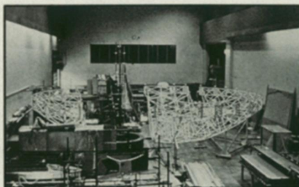
Support for ten-meter mirror for millimeter-wave astronomy is provided by prefabricated metal trusses.
