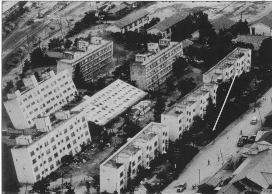
Liquefaction: Buildings in Niigata, Japan, sank into ground intact in 1964 quake.
