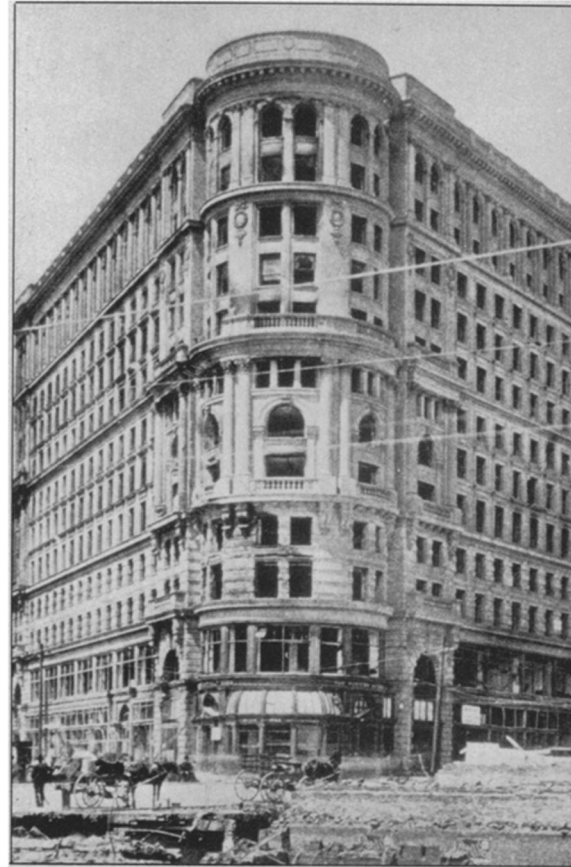
Steel and mortar building that withstood the San Francisco quake and still stands.
