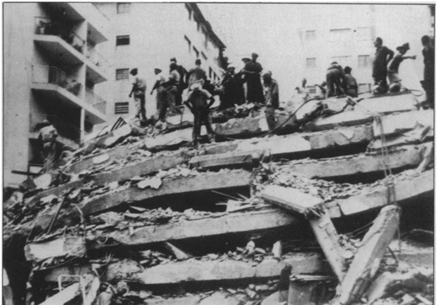
Caracas apartment building with concrete pillars that "pancaked" in 1967 quake.
