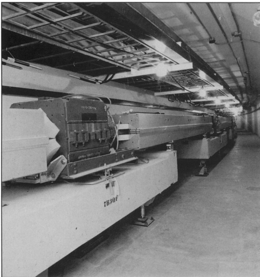
This view of the colliding beam underground shows bending magnets in PEP's tunnel.
