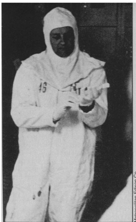
Suited up to inspect damaged TMI plant.
